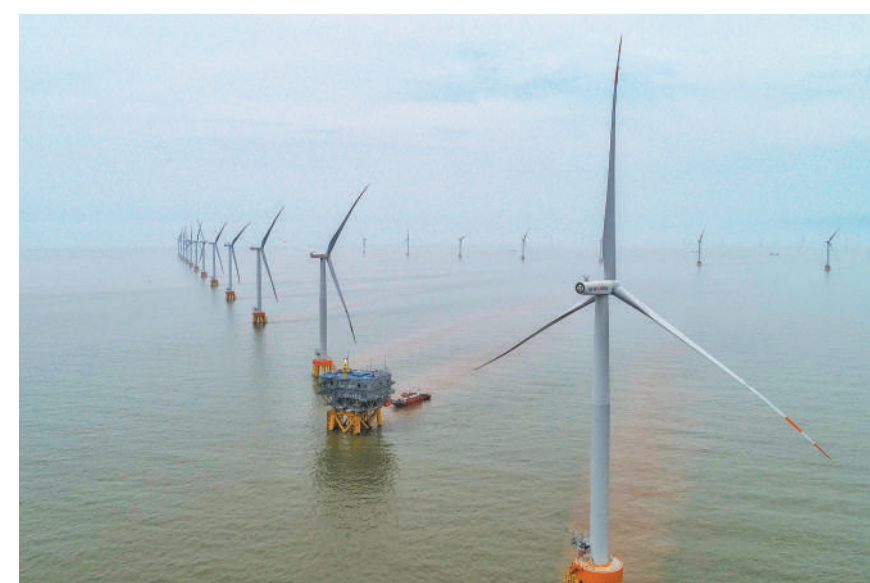
Zhejiang's largest offshore wind power farm in Zhoushan city. (PHOTO: XINHUA)
